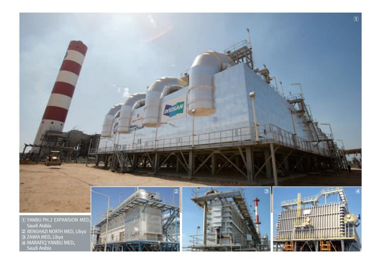
With advanced technologies in scale control and material selection, Multi-Effect Distillation (MED) is now playing a major role in large-scale desalination projects in addition to its traditional application for industrial captive use.
