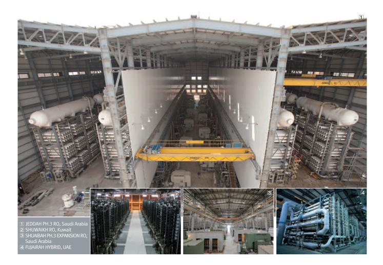
Reverse Osmosis (RO) is a widely-adopted process in which pressure is applied in order to filter salinity from seawater through membranes as opposed to utilizing steam in thermal processes such as MSF and MED. This allows the RO process to have a broader range of applications beyond seawater desalination.
