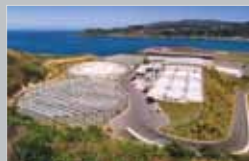
Moa Point Wastewater Treatment Plant /21
