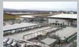
Ringsend Sludge Treatment Plant Extension /23
