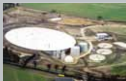
Lowestoft Wastewater Treatment Plant /20
